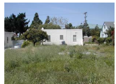
Rear of Old Bldg.
